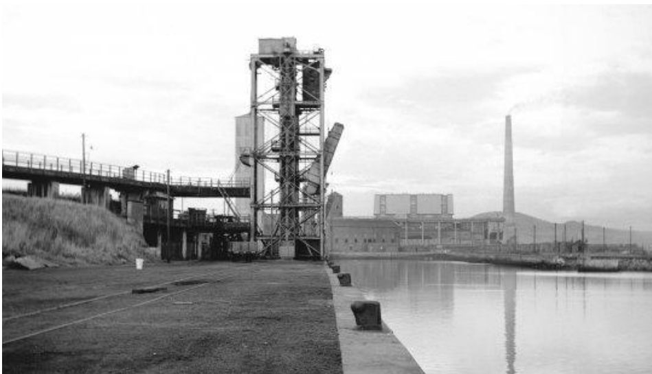
Methil Harbour View from SW showing coal drops with Methil Power Station in the background, 1967. https://canmore.org.uk/collection/610173
