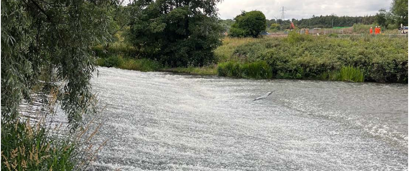
The River Leven at the Kirkland Dam. August 2023
