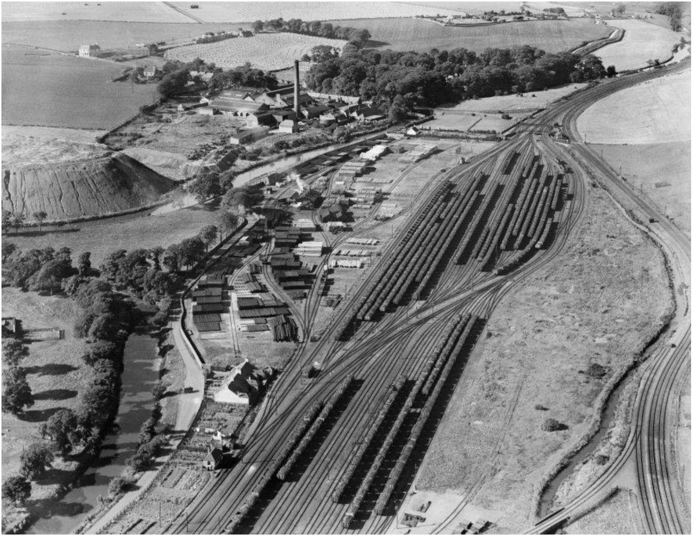
Railway Works on the right-hand side of the photograph and Leven Foundry on the other side of the River. The wood area is the site of the Kirkland House and gardens. The Kirkland Mansion should be located at the left of the foundry. Alexander Bruce and Co. Telegraph Pole and Railway Sleeper Works, Leven. Aerial Photograph. 1932. https://canmore.org.uk/collection/1257434
