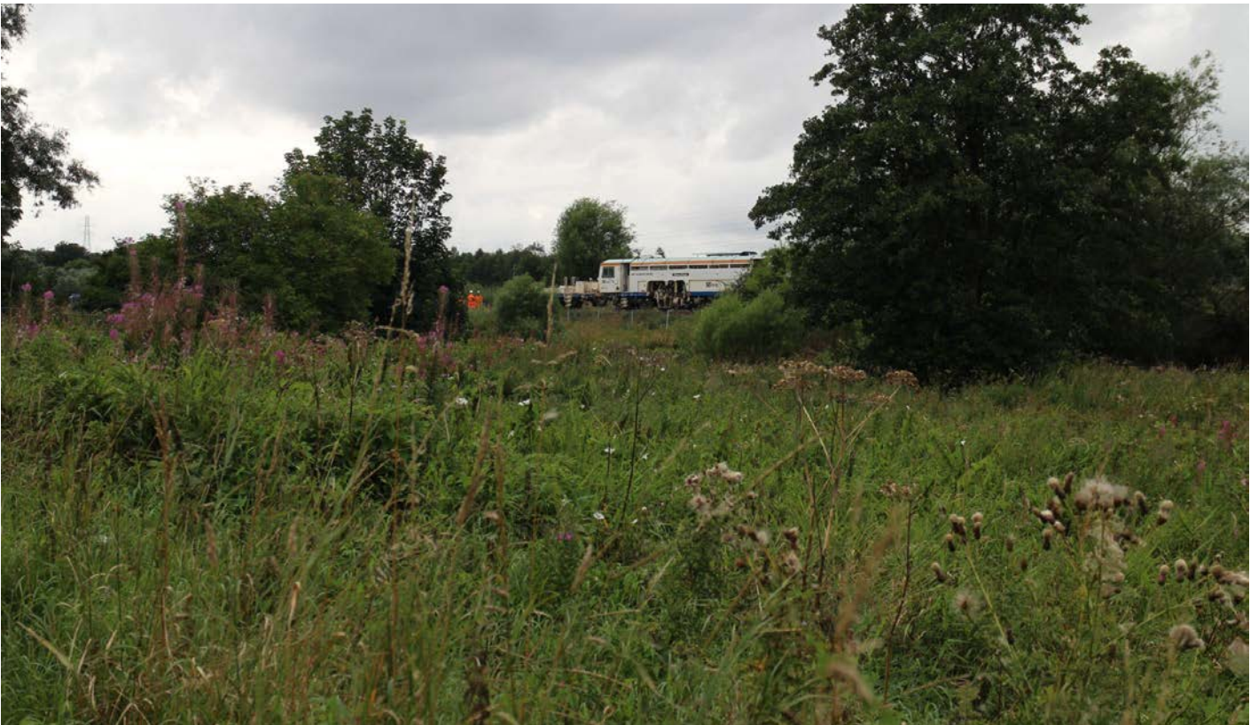
Ongoing work in the River Park to reinstate the rail line, August 2023, icecream architecture.
